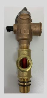
Remove Thermostatic Mixing Valve from the hot water outlet. Pre assemble the pressure relief valve and mixing valve as Pictured
