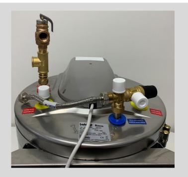
Mount the pre assemble parts onto the hot water outlet of the hot water system.
